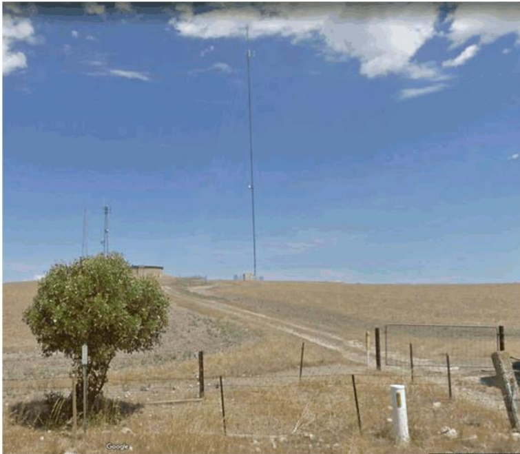
Photo of Towers
