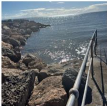
Figure A24: Showing angle of breakwater, not exactly adjacent to ramp this area silts up
