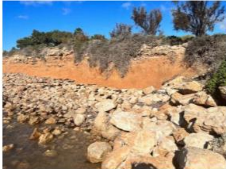
Figure A6: Erosion fronting car park
