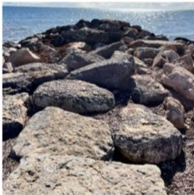
Figure A28: Mid section of breakwater
