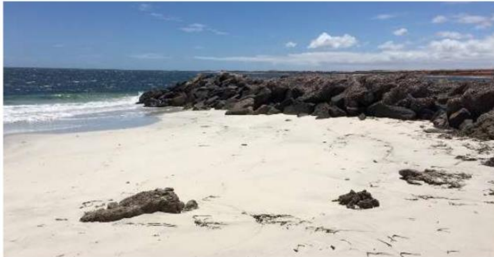
Figure 3: Sediment accumulation (saturation) on south-western side of breakwater (Progress Association 2020)
