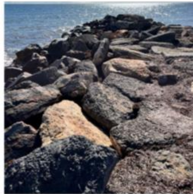
Figure A29: Mid section of breakwater
