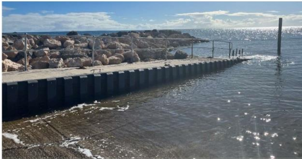
Figure 2: Concrete finger jetty at Balgowan boat ramp
