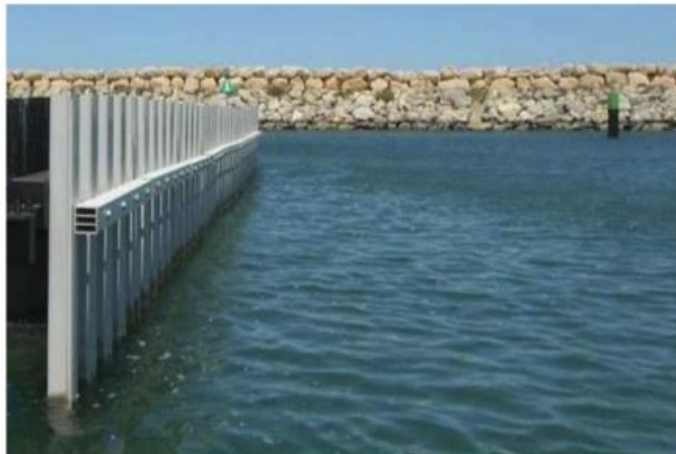
Figure 12: Example wave screen at Mindarie Marina (Chen et al, 2015)
