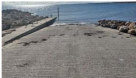
Figure A21: Boat ramp at rising tide
