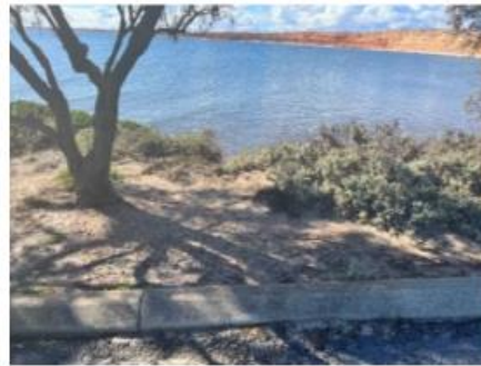
Figure A9: Edge of carpark 2m from erosion pinch point.
