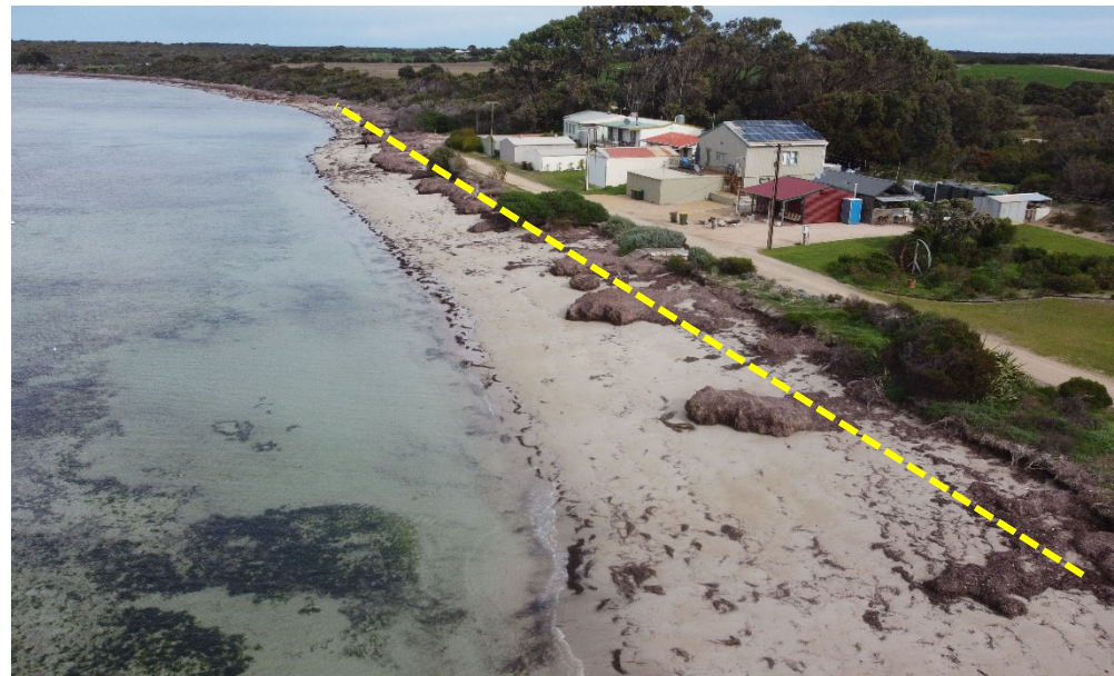
Figure a. The shoreline is rotating (eroding in the west, accreting in the east). The small dune system, which is higher than the road, is being eroded away along Mud Alley. The road is at risk of erosion on the west, and increasing inundation. Two electrical poles are subject to minor inundation at their bases.
