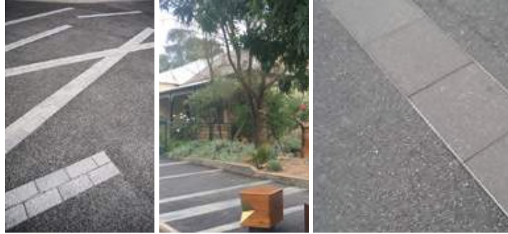
Bitumen with feature paving
