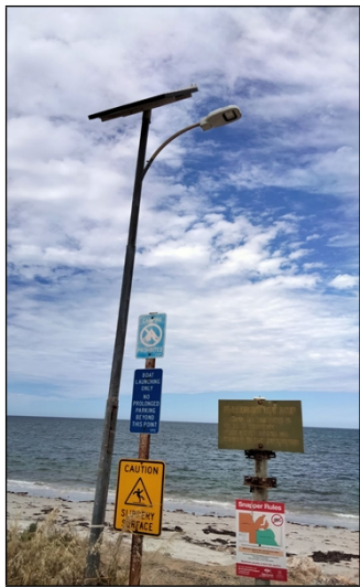
Boat ramp light
