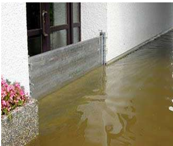
Figure 3:5 Flood diversion/ protection method for dwellings
