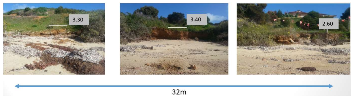
Figure 2:9 Backfill will be required behind the proposed line of rock revetment
