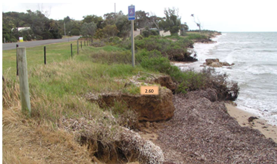
Figure 2:10 Backfill behind rock revetment – sections 1.c and 1.d
