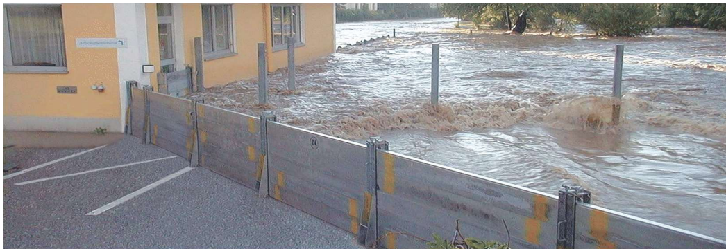
Figure 3:5 Flood diversion/ protection method for dwellings
