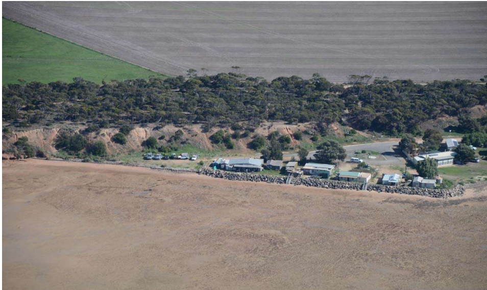
Figure 4:7 Rock armouring to six dwellings on the south end of Port Clinton.
