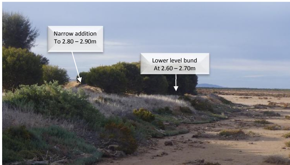
Figure 4:5 Existing sea-flood protection – earthen bund encircling caravan park
