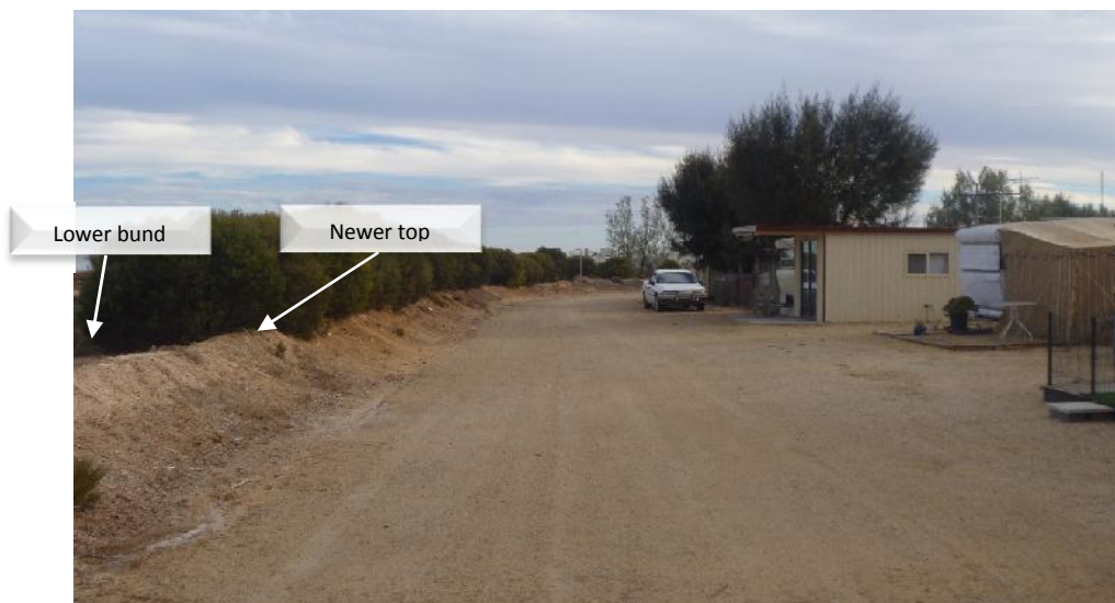
Figure 4:6 Existing sea-flood protection – earthen bund encircling caravan park
