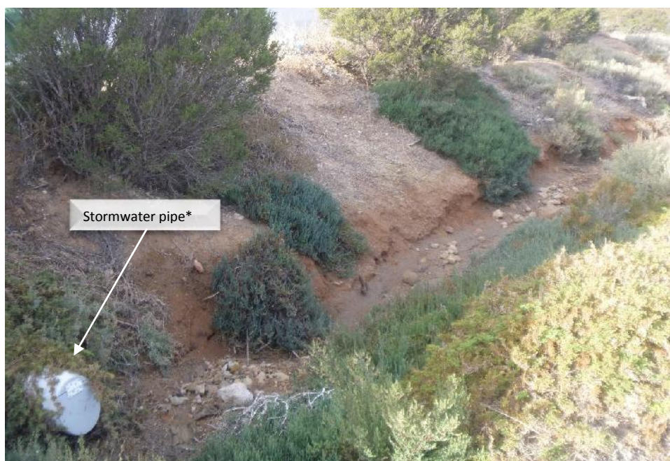
Figure 4:10 Minor erosion of the caravan park bund due to stormwater flows
