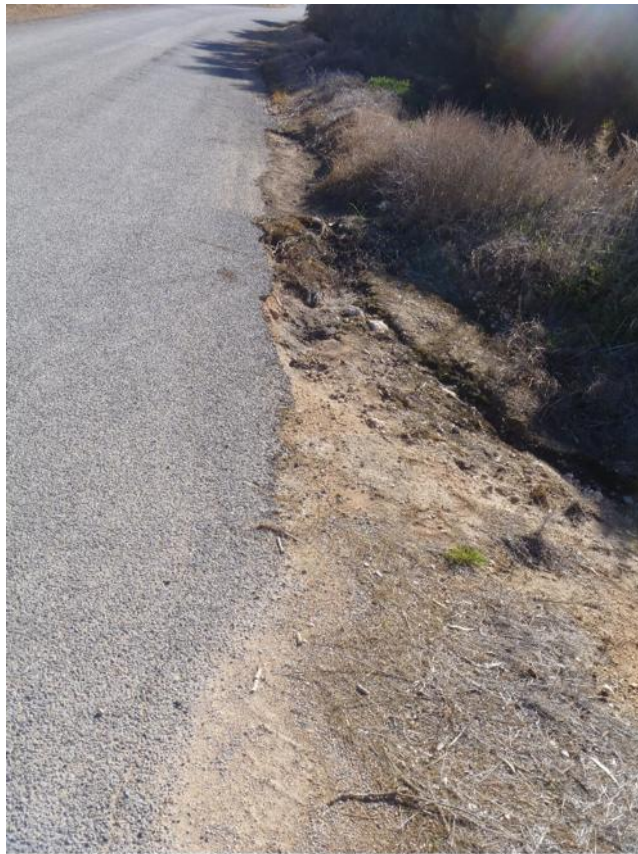
Figure 4:9 Evidence of stormwater erosion at the causeway entrance adjacent the caravan park bund
