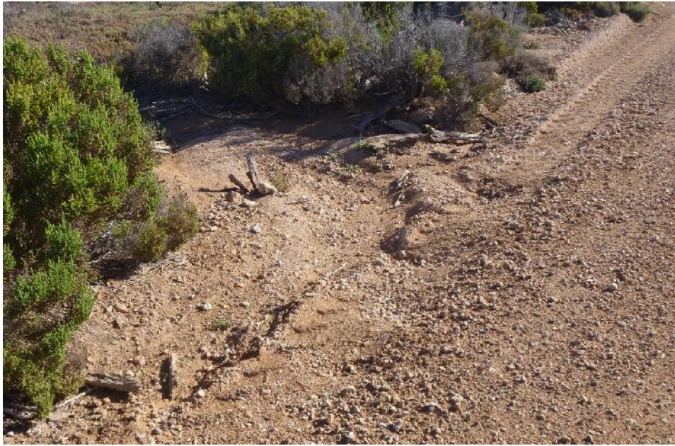
Figure 4:16 Example of erosion on west side of Price boat ramp causeway
